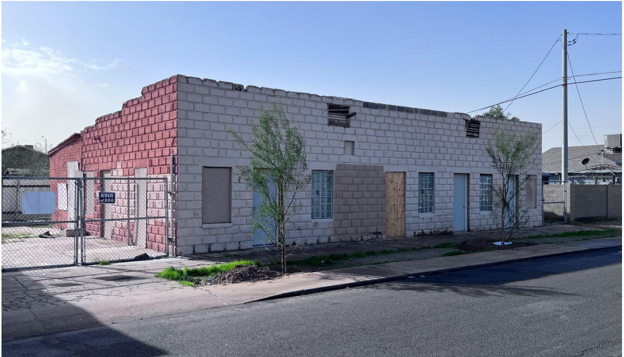
Photo 4. View of north façade of concrete block fourplex, looking southwest from Tonto Street. Photo date: 1/11/2024.
