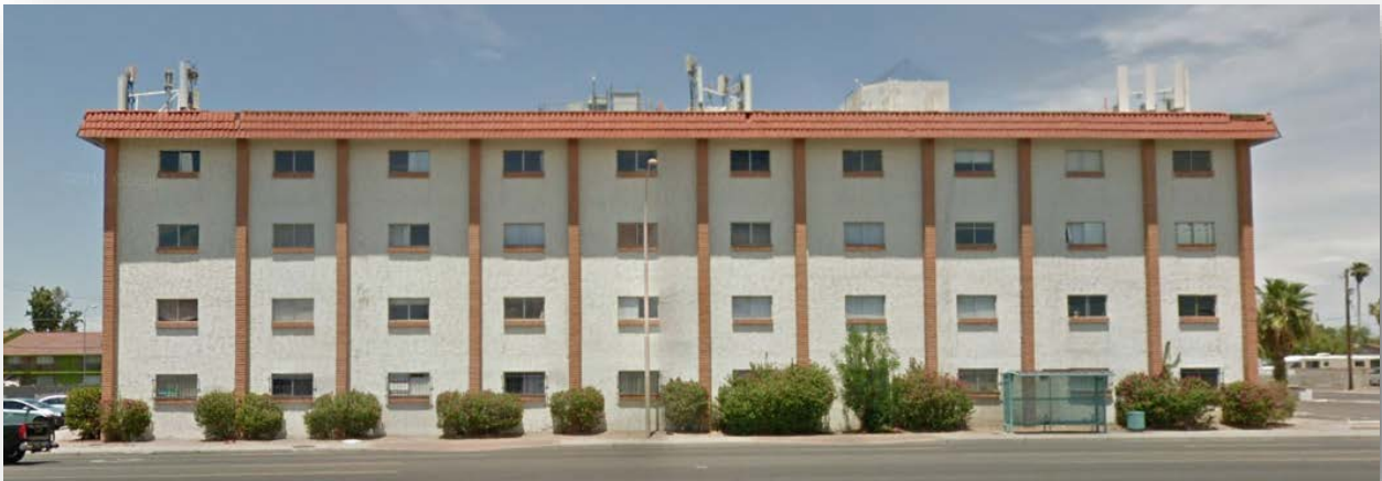
Existing Building Façade Facing McDowell Road
