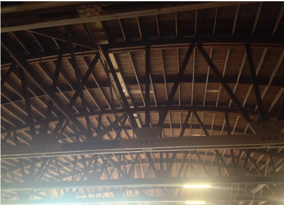
2016 - Interior view - original wood trusses present and recently repaired
