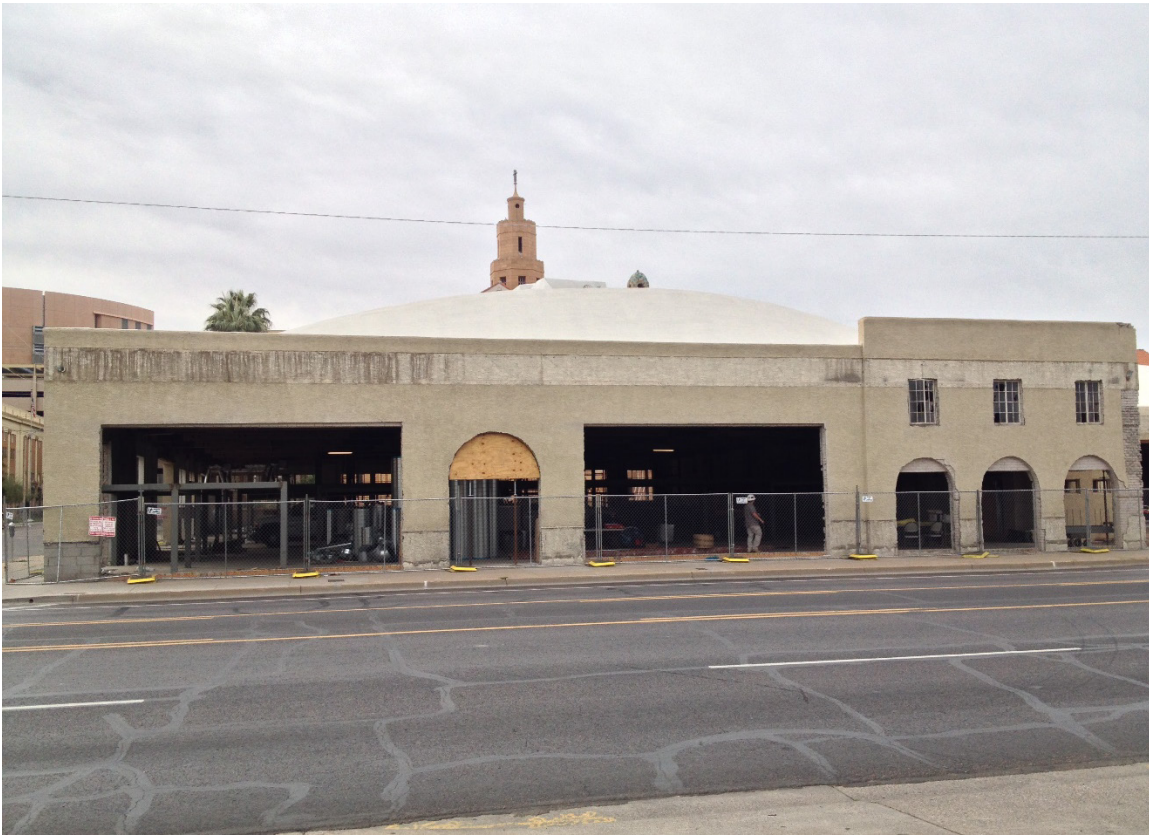
2017 - Exterior view – work in progress to restore historic appearance
