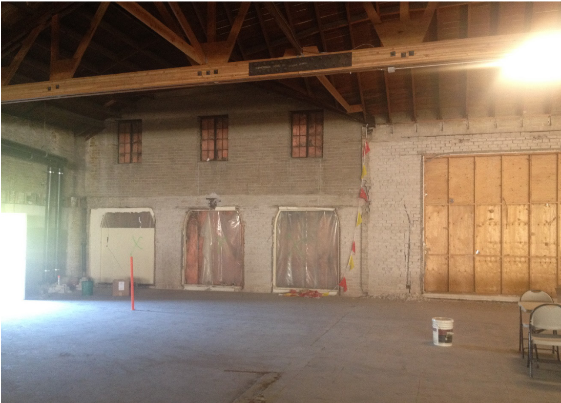
2016 – Interior view - original steel casement windows present
