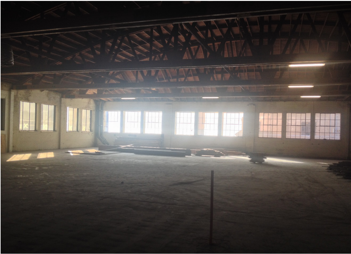
2016 - Interior view - original steel casement windows present
