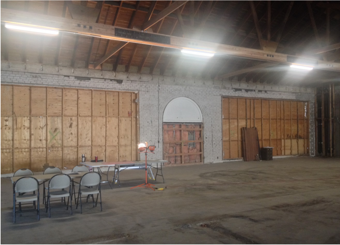
2016 - Interior view - original storefront openings discernible
