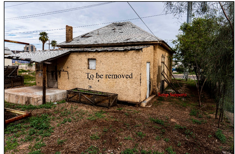
Photo 4. Western facade, looking northeast.
