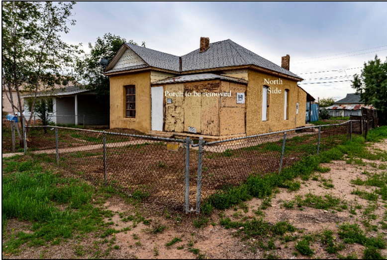
Photo 1. 816 S 3rd Avenue, looking southwest
