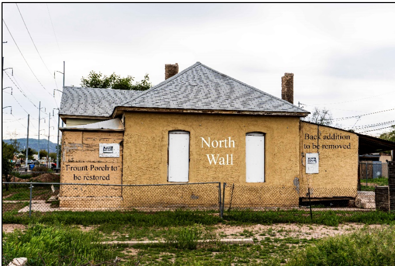
Photo 3. Northern facade, looking south.
