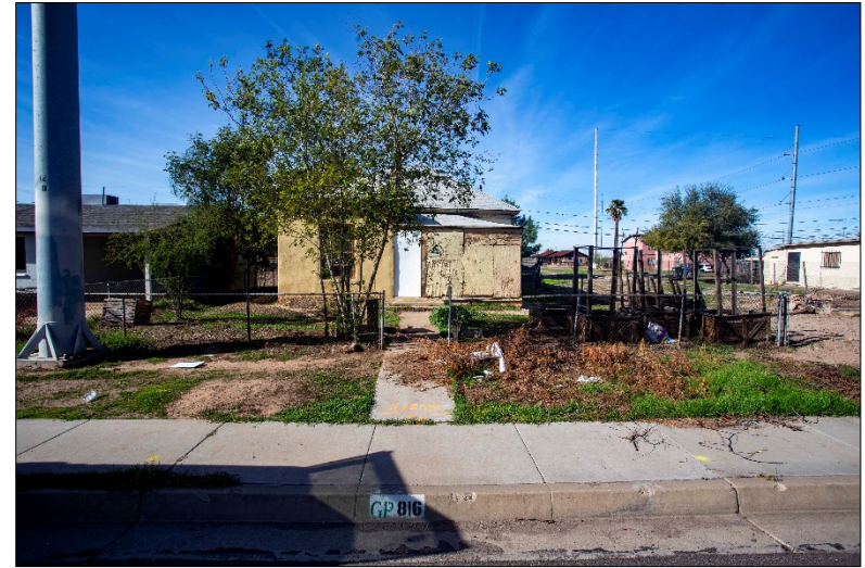
Photo 2. 816 S 3rd Avenue front facade, looking west
