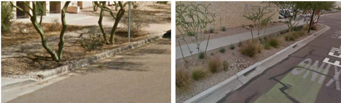
Bioswales reduce runoff and pollution by storing, absorbing and naturally treating stormwater at its source.
