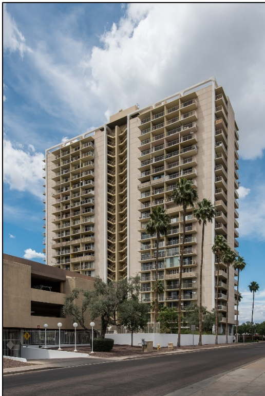
Photo 3. South elevation, with parking garage at lower left, looking northwest.
