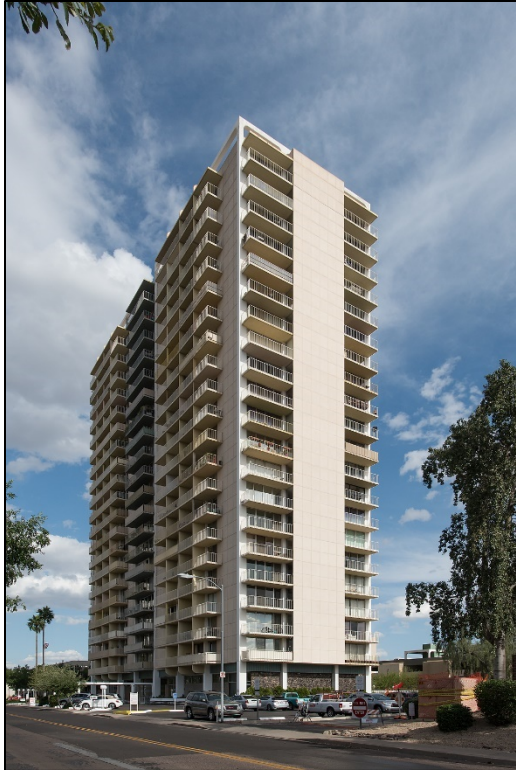
Photo 1. Main north façade and the west elevation, looking southeast.
