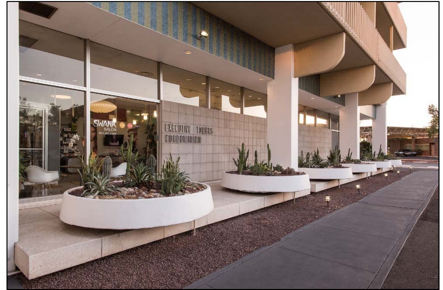
Photo 14. Base of north elevation, main façade, looking southwest.
