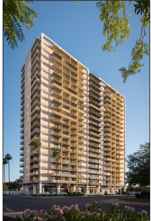
Photo 2. Main façade, with a portion of the east elevation, looking southwest.
