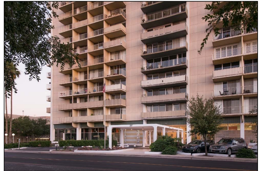
Photo 16. Base of north elevation, main façade, showing porte-cochère and entrance, looking southeast.
