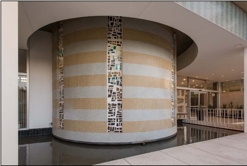
Photo 13. Base of first floor, curved projection with mosaic bands and stained glass, looking southwest.
