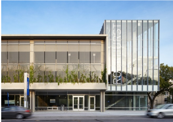
Example: Well integrated screening for parking structure
