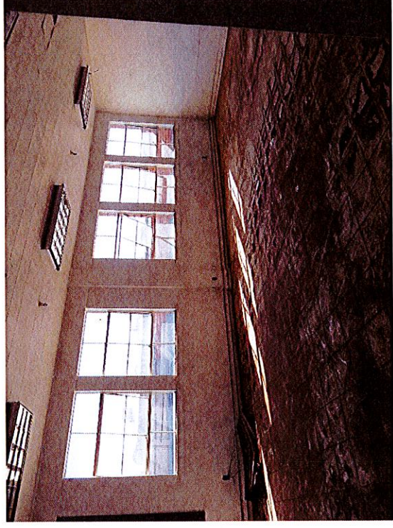
16. Interior second floor east wall, camera facing southeast.
