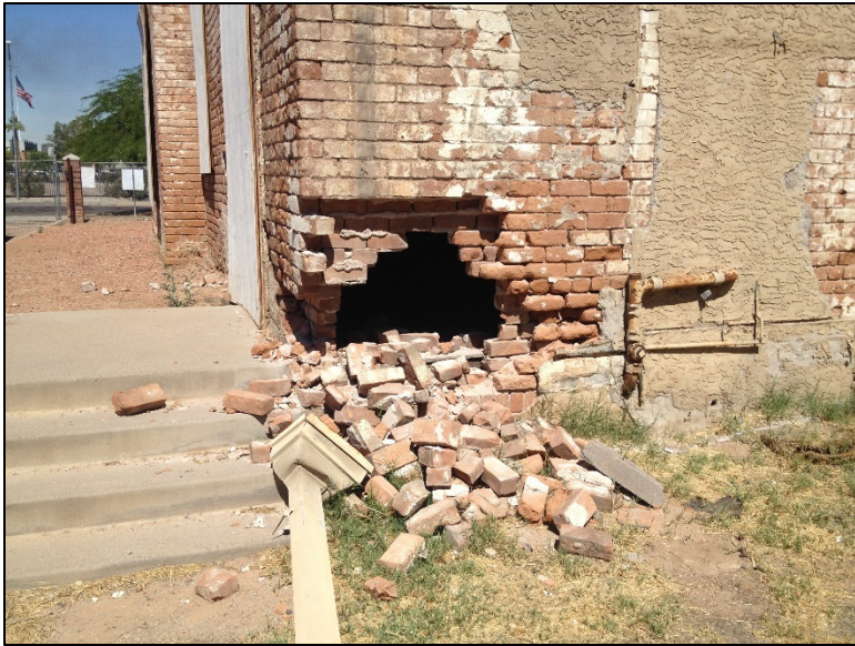
Photo 13. Close-up view of southeast corner of house, looking west from rear yard.
