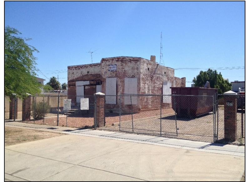
Photo 2. View of subject property, looking northeast from 4 th Avenue.
