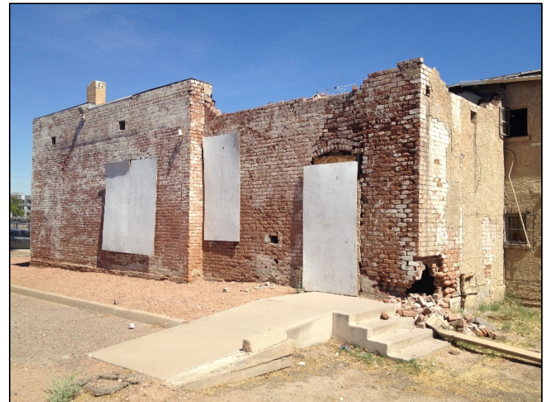
Photo 12. View of subject property, looking northwest from adjacent lot to south.
