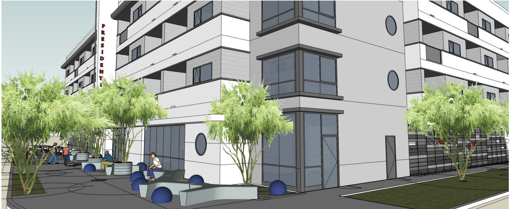
View from the Southeast corner of Washington Street and 11 th Street
