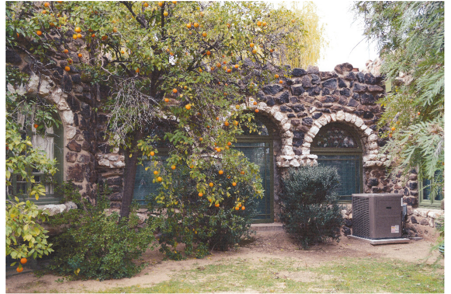
2. Front view of house, looking northeast from front yard.
