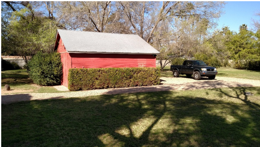
7. View of accessory building, looking west from rear yard.
