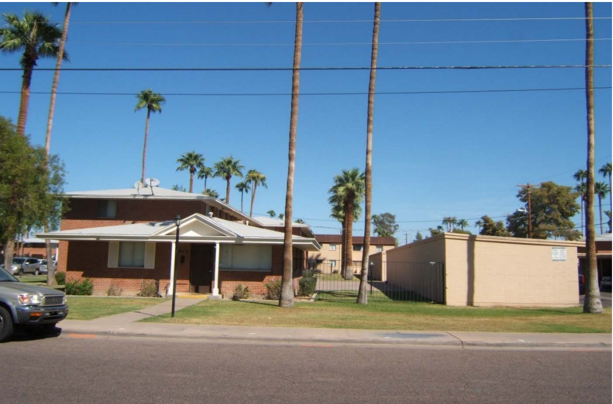
Photo 22: Cottage apartment with adjacent carport (City of Phoenix, 2018)
