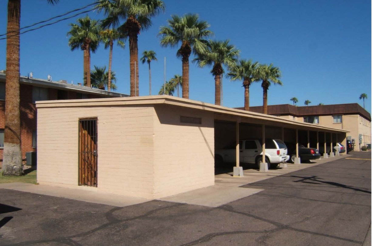
Photo 23: Rear alley carport structure (City of Phoenix, 2018)
