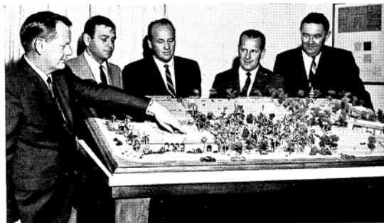
Robert Marsh (left), assistant secretary of Harsh Building Company, owners of Park Lee Alice Apartments, 4702 No. 15th Ave., explains miniature replica of the project's 4½ acre recreational facilities to: (left to right) Jerry Bialac, former owner of the development; Ray Thornborough, State Registrar of Contractors; Mayor Milton Graham; and City Manager, Robert Coop.
