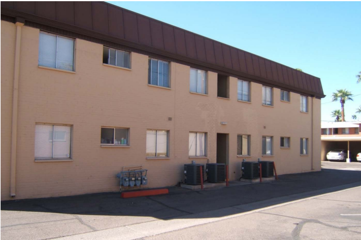
Photo 26: Rear façade of apartment building
