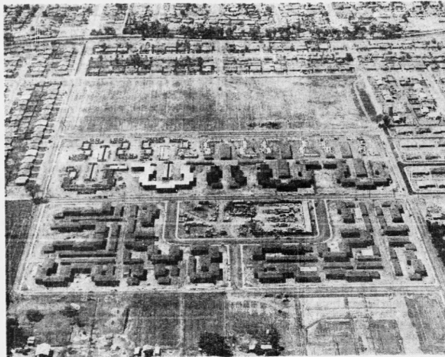
Progress Report First apartments in the huge Park Lee Alice project are to be ready for tenants in June. In the picture above the shopping center foundations at the corner of 17th Avenue and Camelback, are seen in the lower right corner. The street across lower part of view is Pierson. The construction yard in center will become a three-acre park. It faces on Highland. The approximately 30 vacant acres at top are owned by corporation and apartments may be built there also. (Aerial Photo, Donn Nobles)
