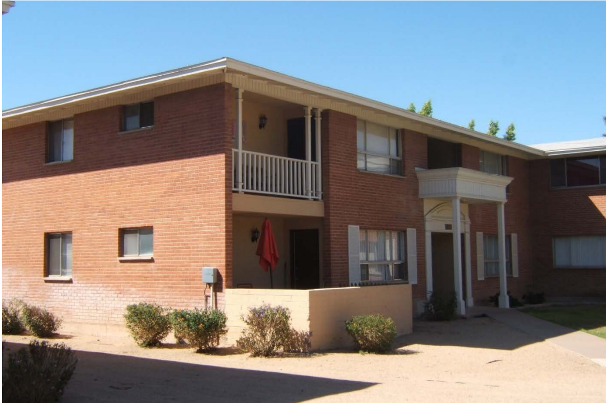
Photo 5. Apartment building (City of Phoenix, 2018)
