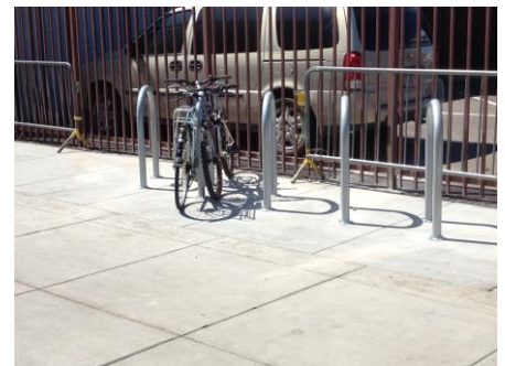
Inverted-U racks allow bicycles to touch the rack in two places, providing stability and allowing the wheels and frame to be secured to the rack.
