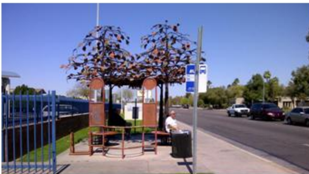
Case Study: Iron tree bus stop installation
