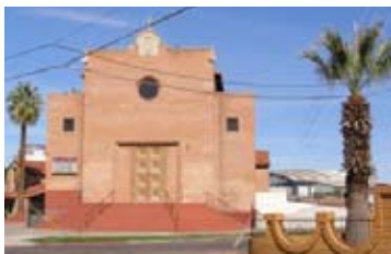
Historic Property 7: St. Anthony's Catholic Church
