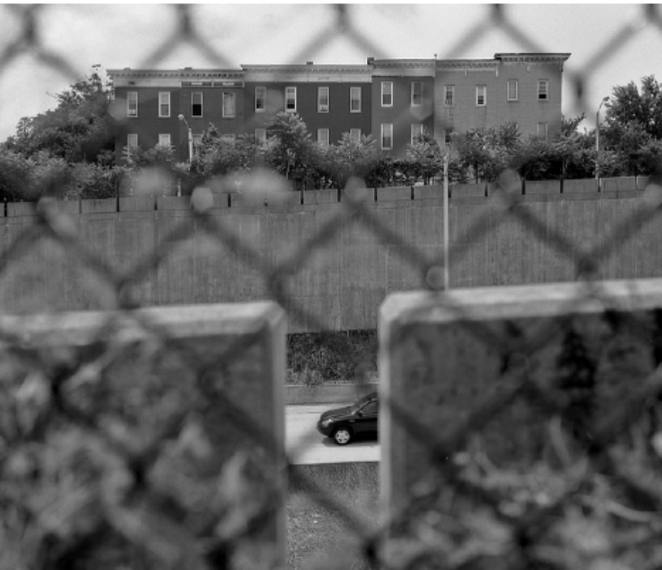
Re-Connect West Baltimore will create safe passage over U.S. 40 that currently divides the neighborhood. Image provided by OST.
