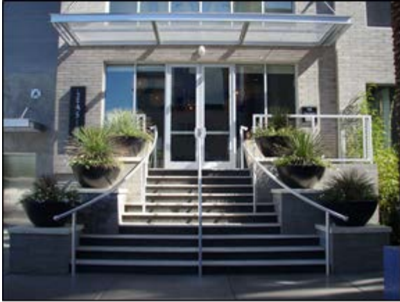
Example of Building Entrance with Elevator Access
