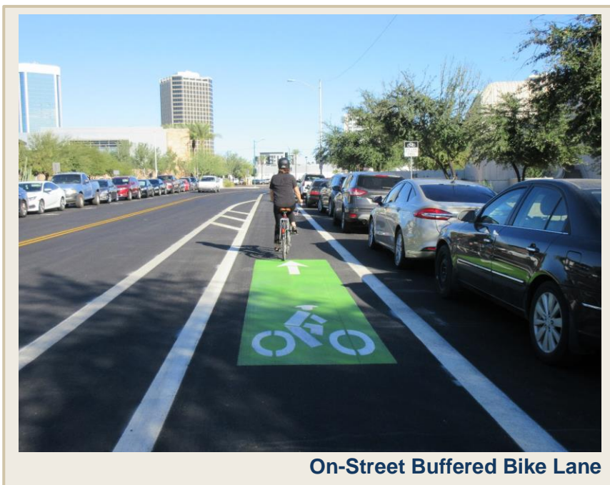
Figure 8.5-2 On-Street Buffered Bike Lane
