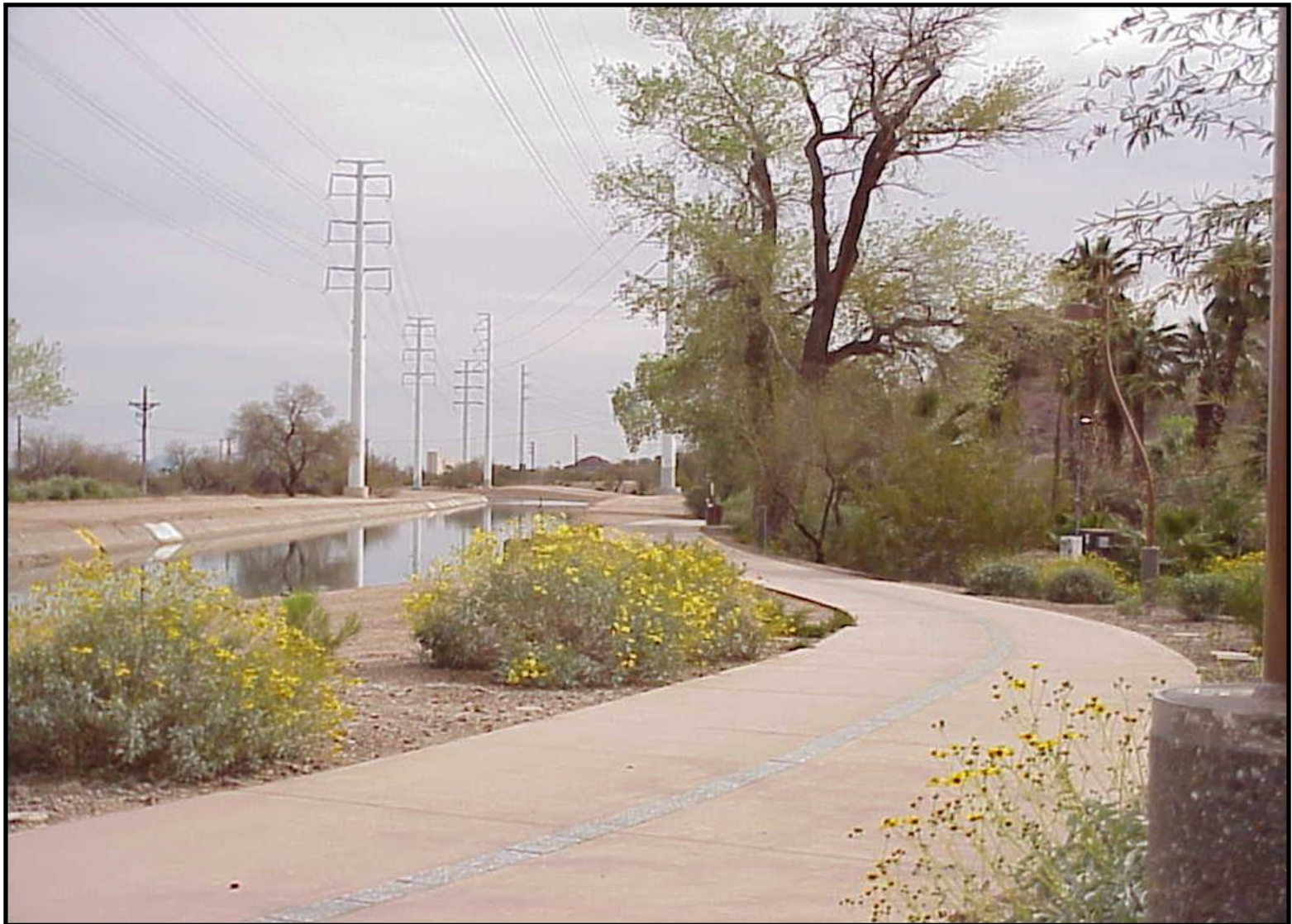
Canal Multiple Use on the SRP Canal System Water 101 July 11, 2012
