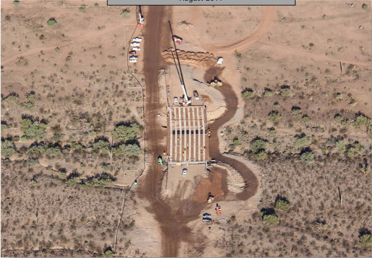
Cave Creek Secondary Wash Bridge August 2011
