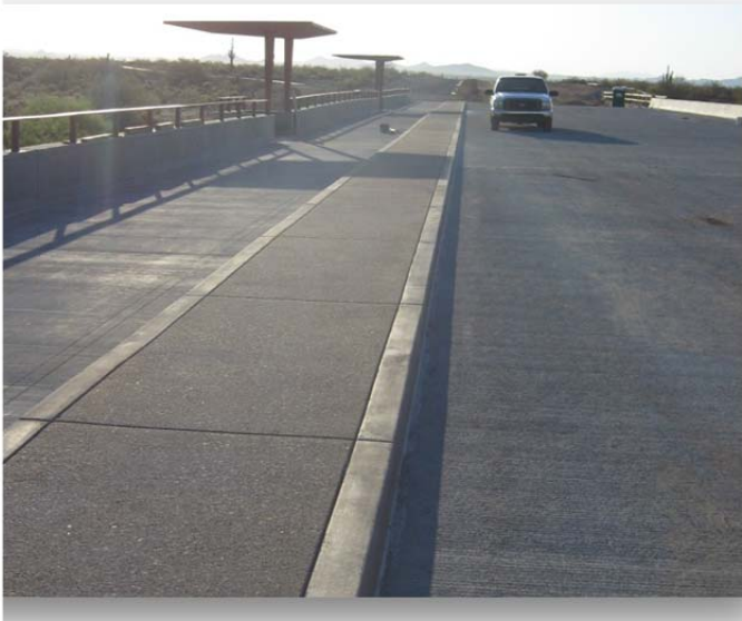
Apache Wash Bridge September 2012
