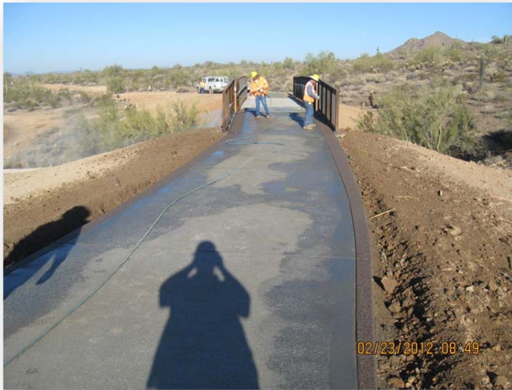
Paseo Path at Pedestrian Bridge Construction February 2012
