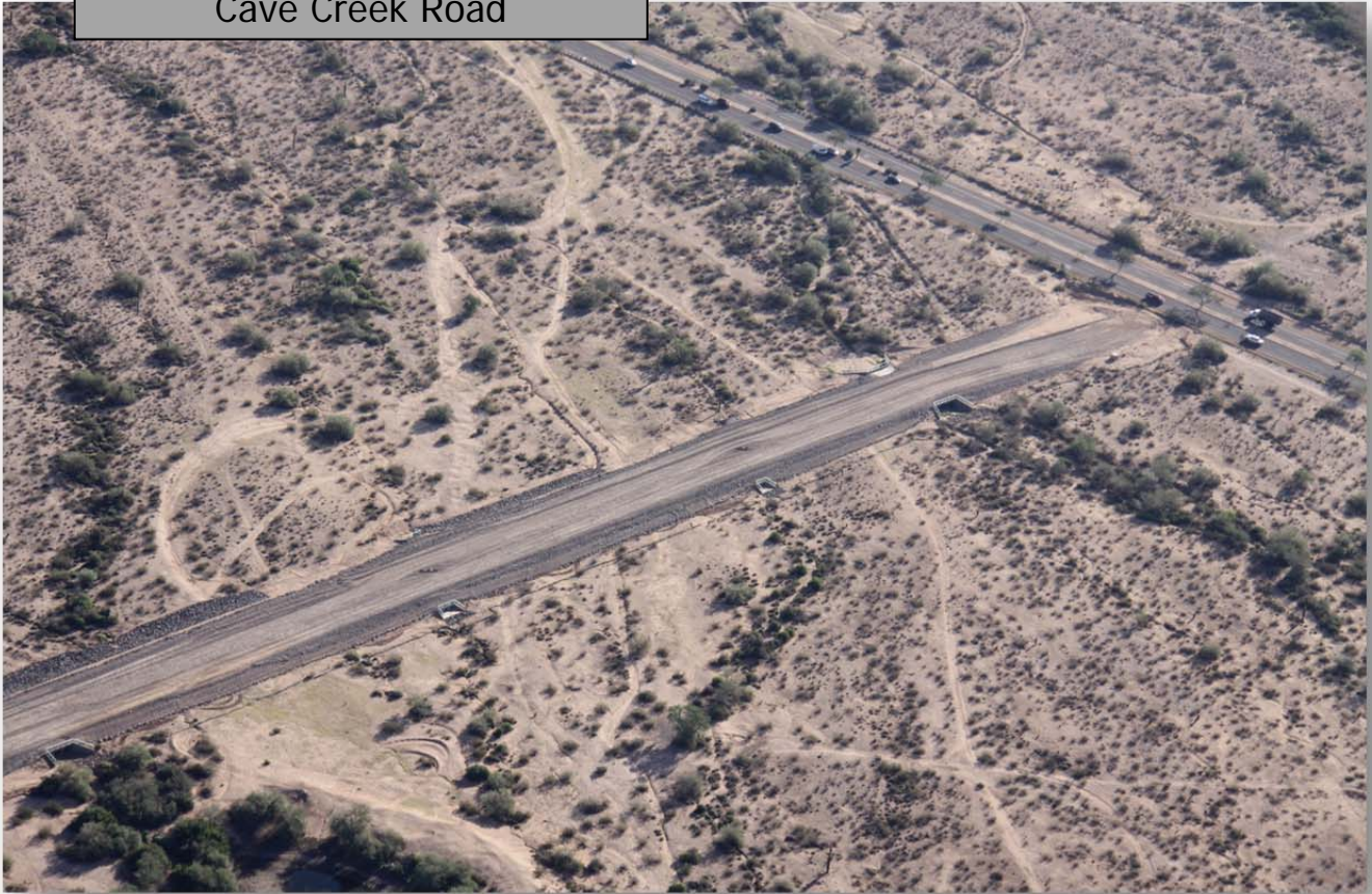
View from Cave Creek Road looking West
