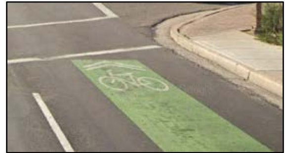
Marked Shared Lane on Fillmore Street
