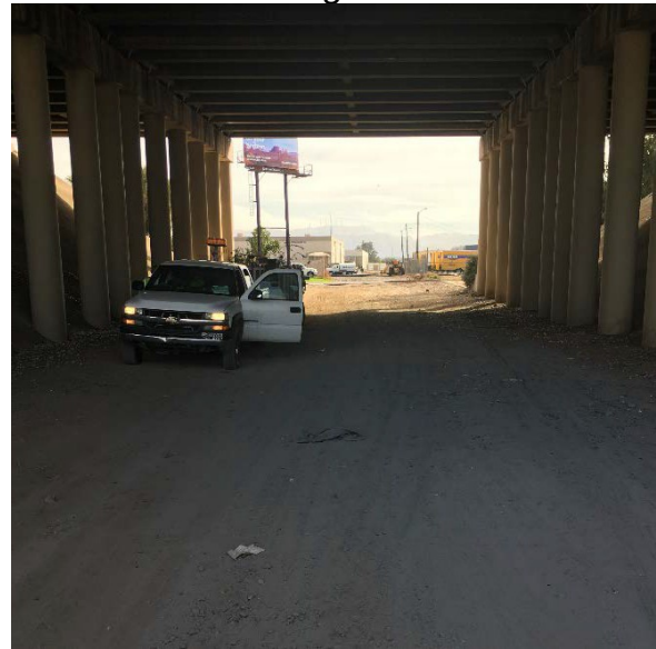
Photo 23 - 3rd St Underpass, I-17, Looking South
