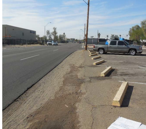
Photo 9 - Buckeye Rd, West of 3rd St, Looking West
