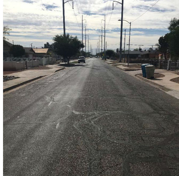
Photo 16 - Hadley St, East of 3rd Ave, Looking East
