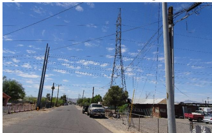
Figure 5-17: Lack of shade along local street
