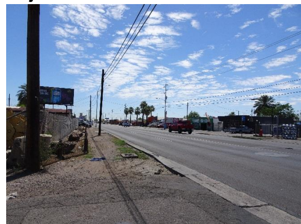
Figure 5-14: Street lighting along major arterial
