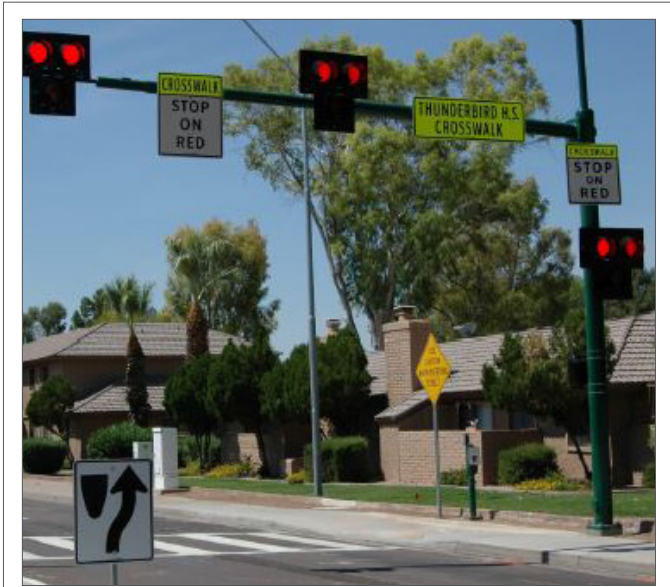
On June 25, 2020, Phoenix's 66th HAWK pedestrian crossing signal was activated at 18th Street and Roosevelt Street. HAWKs make streets safer for people who walk, bike and drive by providing clear alerts when people intend to cross the road.
