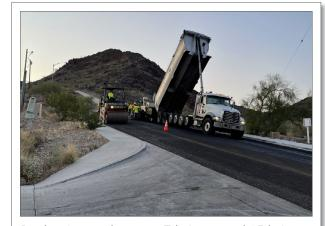
Dunlap Avenue between 7th Street and 15th Street received mill and overlay work, which includes removal of the top layer of a street (milling) followed by laying new asphalt (overlaying).
