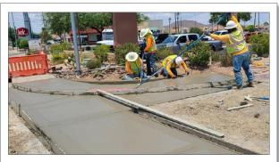
Crews install curb ramps to provide a safe route that people with disabilities can use to transition from a curbed sidewalk to roadway and vice versa.
