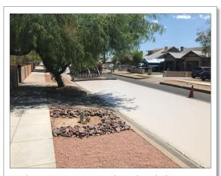
Cool pavement is a water-based asphalt treatment that is applied on top of the existing asphalt pavement.
