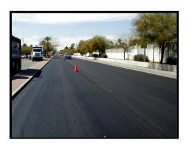
Microseal is similar to slurry seal in appearance and application, but used on major and collector streets. It uses larger aggregate (coarse sand) and a polymer-modified emulsion. The modified emulsion sets very fast and lets the material withstand heavy traffic loads. It is typically used on newer arterial and collector streets with minimal cracking and patching to replace lost fines and provide a new wearing surface.
