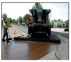
Slurry seal is a mixture of emulsified asphalt and fine aggregate (i.e., sand) applied to local streets to replace the loss of fine aggregate, protect the original surface, and provide a new wearing surface. To be most effective, the treatment should be applied to low volume streets with little cracking, usually to pavements less than ten years old.
