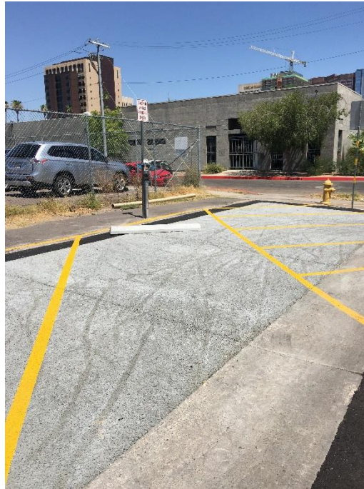
1st Street and Buchanan – Back-in parking with eight (8) pervious-concrete parking stalls.
